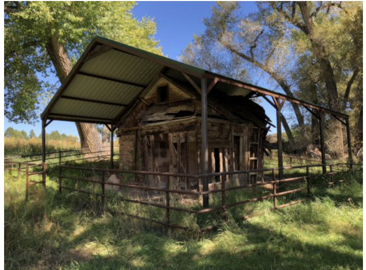
The historic Barlow House on Stonewall Creek Ranch
