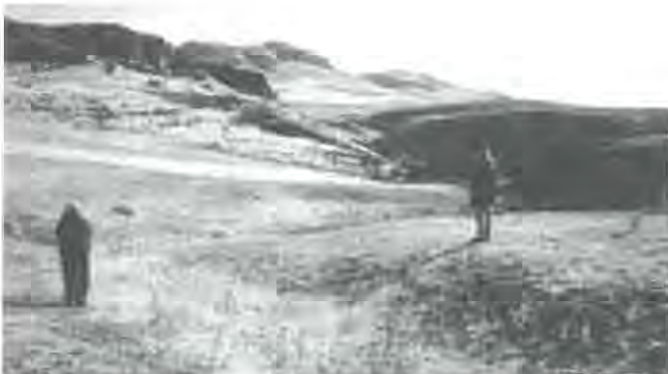
Kelton Ruts from Canyon Creek. Wally Meyer, right, and Jim McGill, left. (Photos by Bill Wilson)
